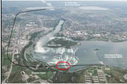
Dam Project, Ontario, Canada
